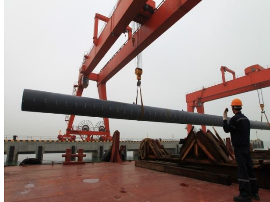
Our own frame cranes for 100m long pipes
